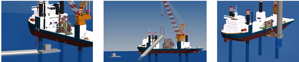
Figure 2: Hook on-, upend - and positioning of pile
