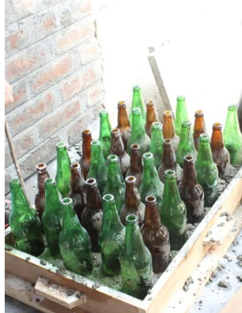
**Figure 5.2:** Construction process in a mould by Mud Hands
