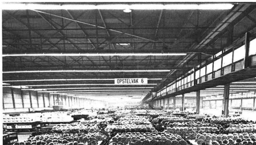
Figure 6.3.1. Typical example of application of hot-dip galvanizing: nearly 10,000 tons of hot-dip galvanized steel have been used for the enormous halls of the Aalsmeer flower market.
