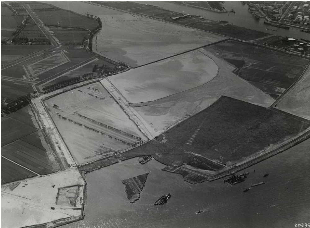
Aerial view of the digging of the second Petroleumhaven, from the northeast, Rotterdam, 1946. Collection of Stadsarchief Rotterdam (SAR), VII-450-01-02-3, 4232
