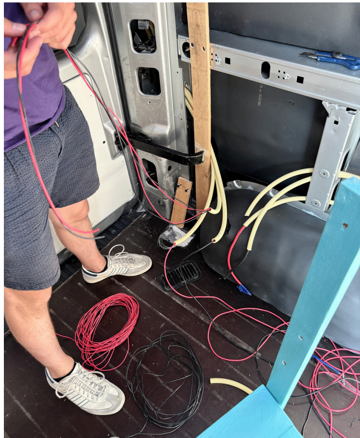
Figure 2.12 Author installing electrical wiring
