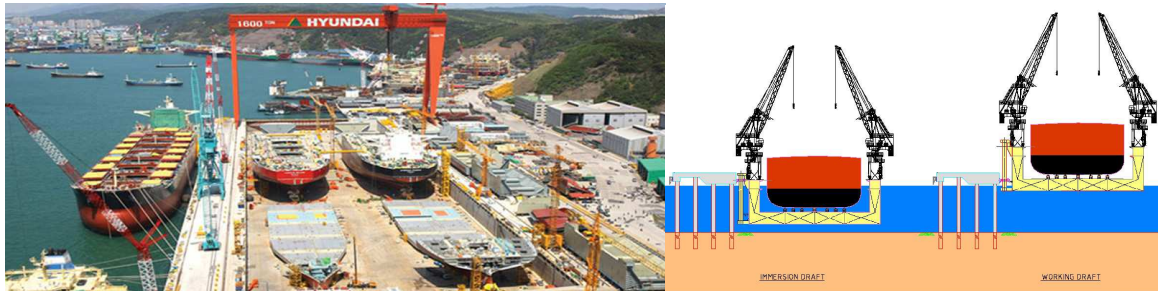
Figure 45 - Dry docks: a) Fixed dry dock (Ulsan, South Korea) b) Floating dry dock principle
