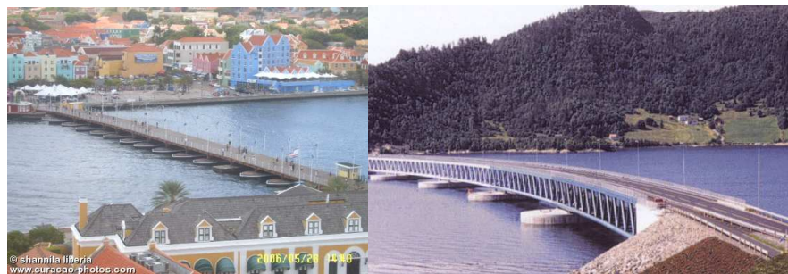
Figure 46 - Floating bridges: a) Queen Emma Bridge b) Bergsøysundet Bridge
