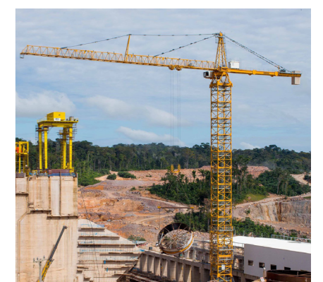
Liebherr heavy load crane (2000 HC 60)
