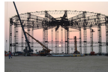
Stageco lightweight modular concert construction
