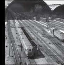
Structural renovation for increased regional and international train traffic
