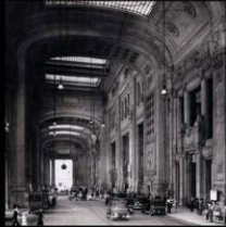
Poor accessibility of the tracks, inadequacy of services
