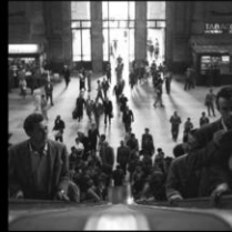
Installation of escalator system to connect the different levels
