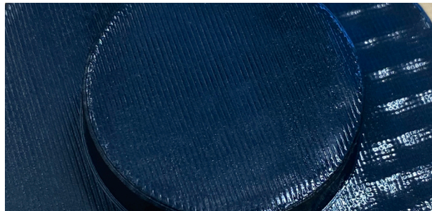
Figure 65: Infill showing after smoothing plastic with a heat gun
