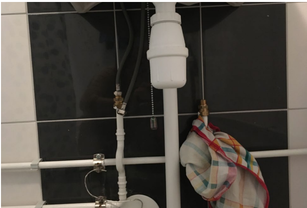
Figure 53. Leakage by installing a flow sensor
