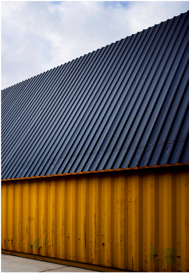
Fig. 6. Corrugated sandwich roof panels and shipping containers (detail).
