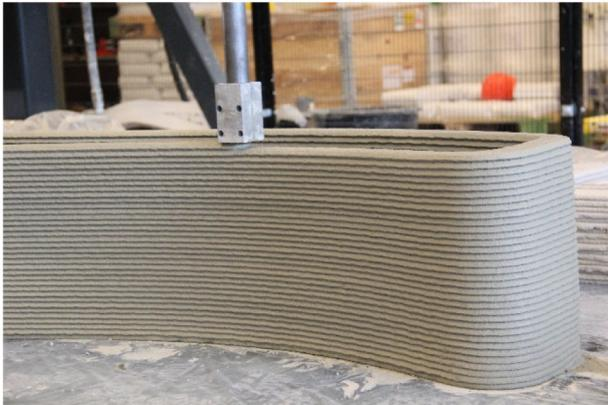
Figure 2.8: 3D printed concrete layers [126]
