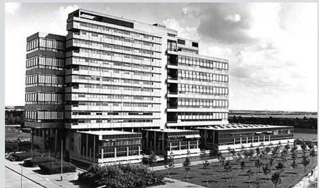
Figure 19: the former Architecture faculty
