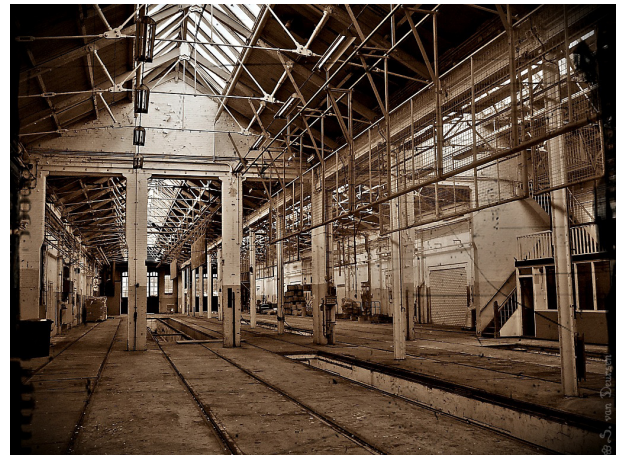
Figure 11: De hallen before redevelopment
