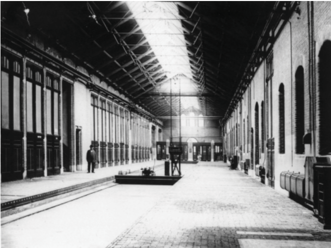
Figure 24: De western tram depot soon after completion
