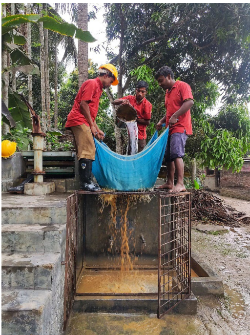
Figure 3: Backwashing procedure in Kolaroa, Bangladesh. Arsenic containing iron sludge is directly disposed into the environment.
