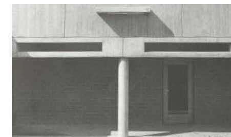
fig 24: The recurring structural elements of the building.
