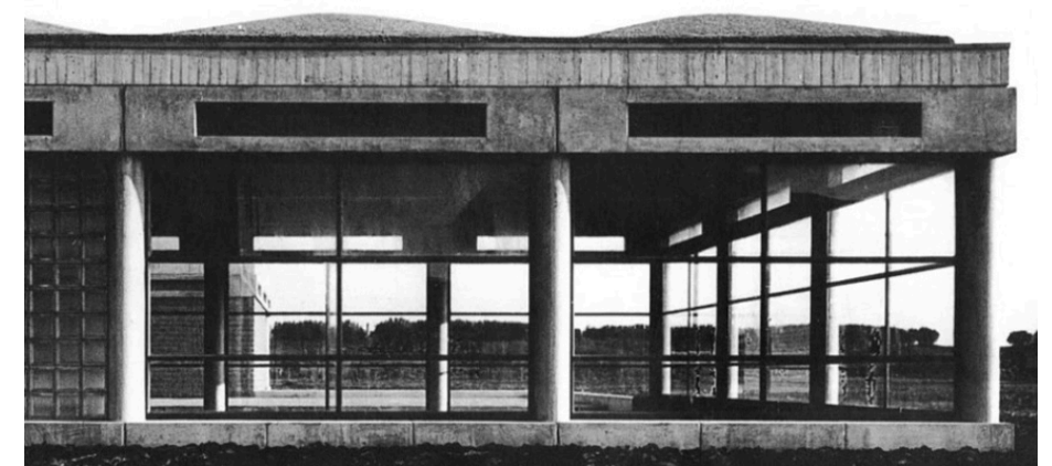
fig 18: Picture showing the elements combined, constructing the building
