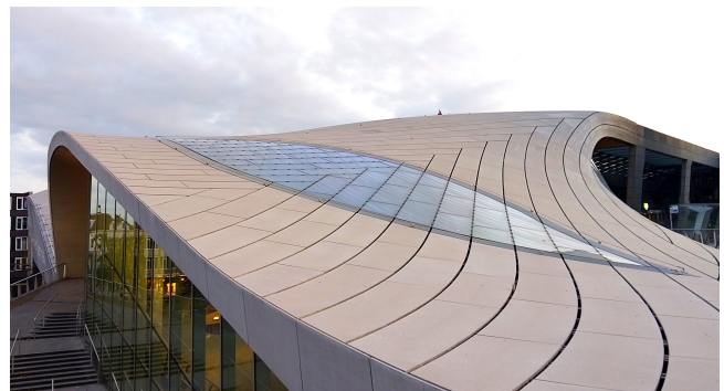
Figure 16: Extending our approach to 2D could allow the reuse of wind turbine blade panels for cladding of curved architectural structures (inspirational illustration: roof of Arnhem Central station).
