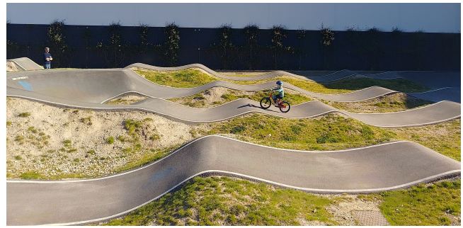
Figure 2: Pumptracks can feature rollers and corners of varied curvature, making them a rich object of study for shape design.
