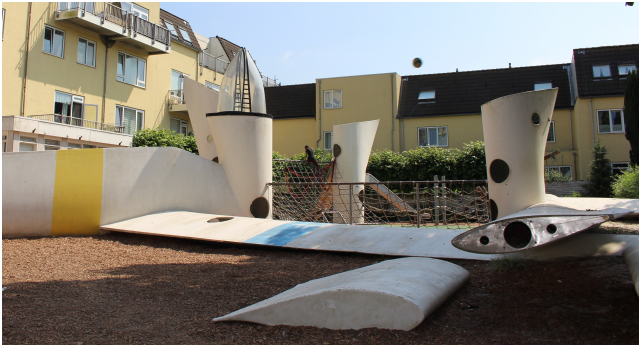
Figure 3: The Wikado playground by SuperUse studios, Rotterdam, illustrates how wind turbine blades can be creatively repurposed as construction elements.
