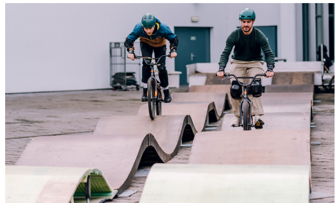
Figure 8: Setup for the pumptrack test event: two parallel tracks, the final rollers made with wind turbine blade panels. Picture by ©Patrick Wetzels, TU Delft.
