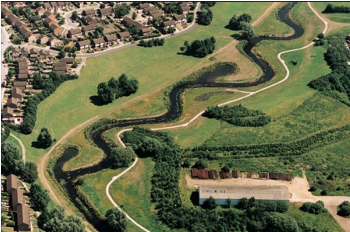
Completed meanders – Summer 1997
