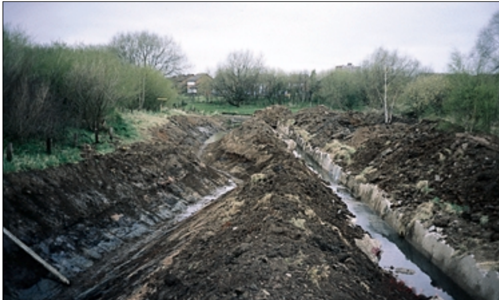
The 'new' Brook being excavated adjacent to the old channel. Spoil stockpiled
