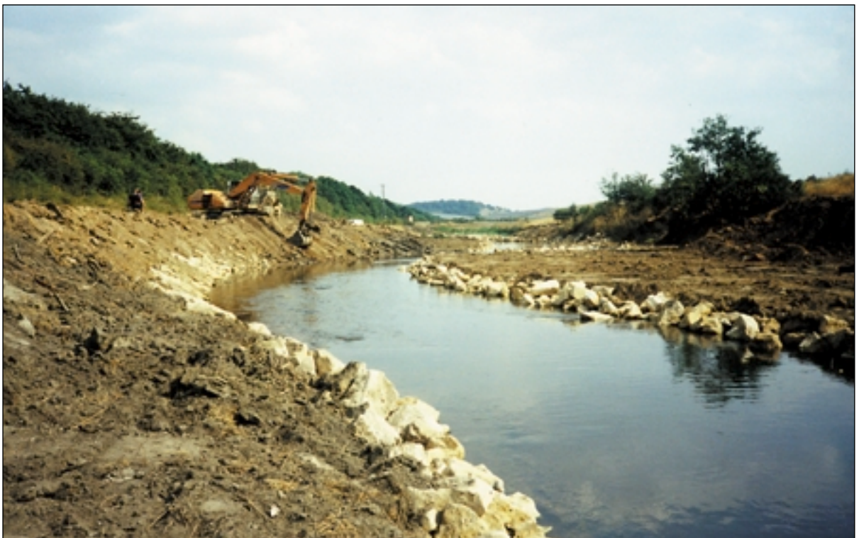
Placement of limestone boulders and berm back-filling
