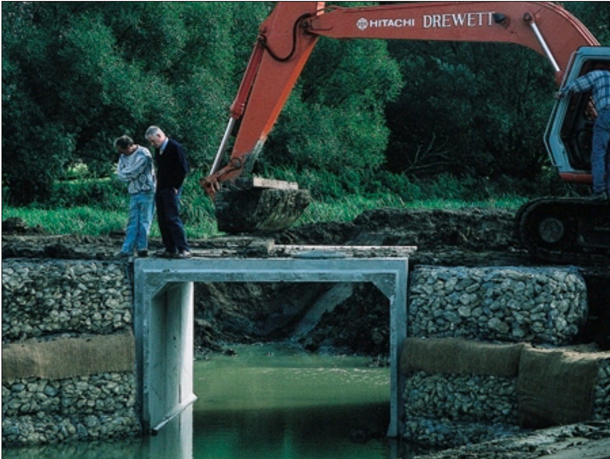
New concrete culvert crossing under construction
