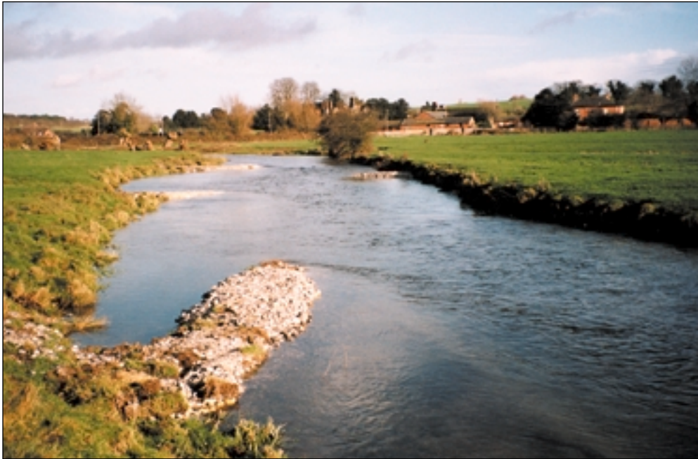
Completed chalk groynes
