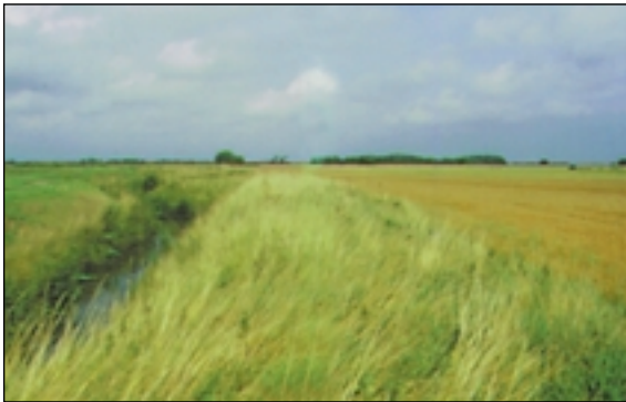
View along the trapezoidal right bank of the Long Eau
