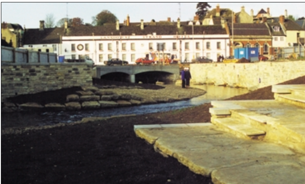
Completion: View of the new river course
