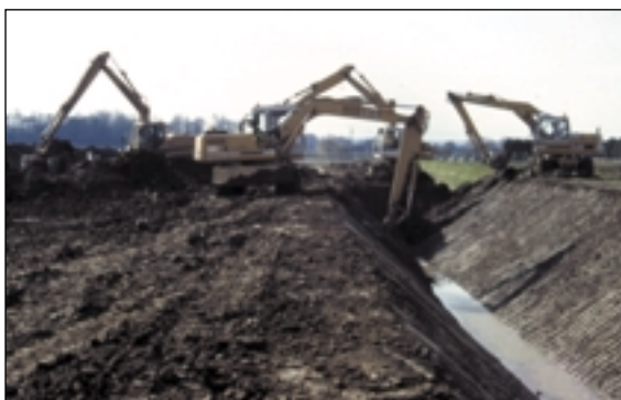
Relocating the IDB drain and set-back floodbank
