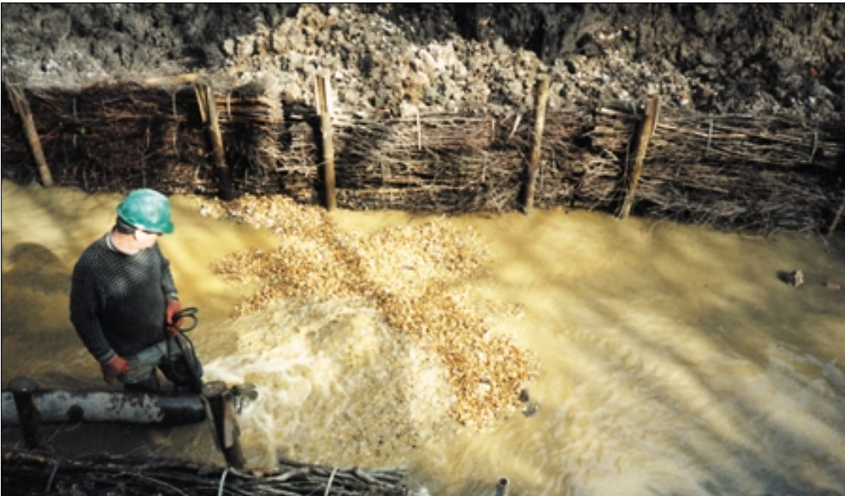
Gravel pumping in operation
