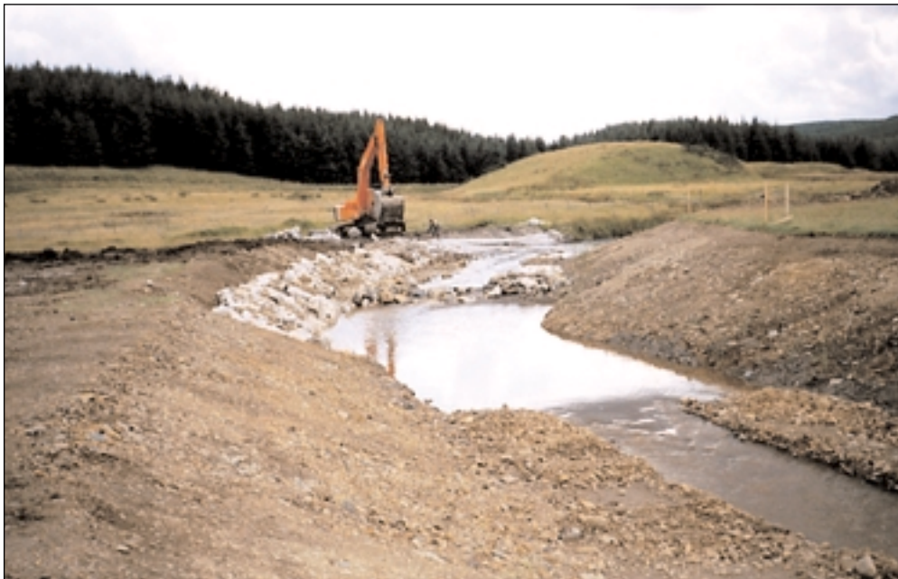
The 'constructed' run-pool-riffle sequence
