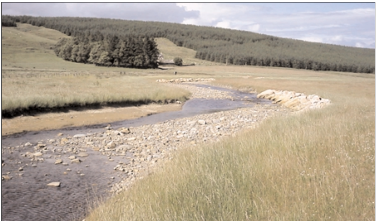
One year on and natural redistribution of in-channel sediments is helping to 'soften' the engineered channel
