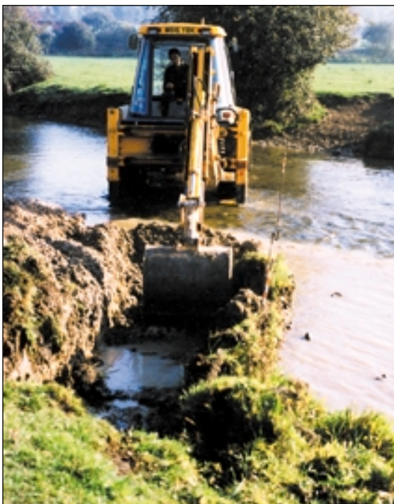
Digging the groyne trench
