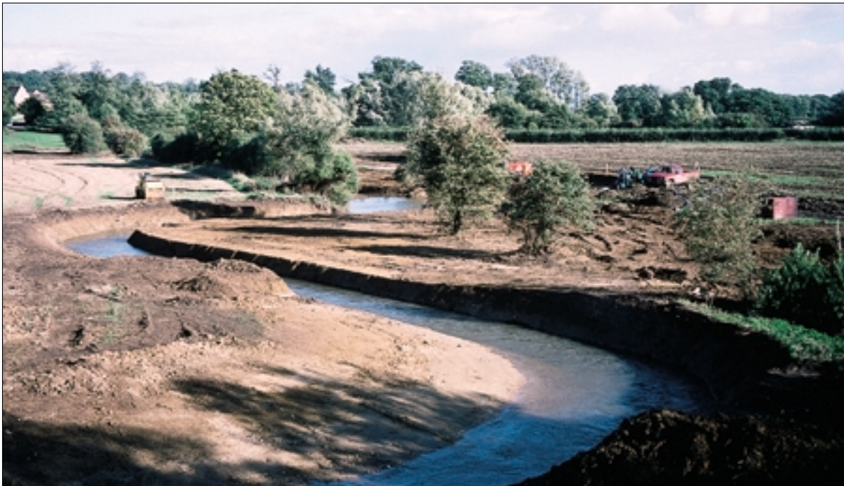
Meanders during construction – 1995
