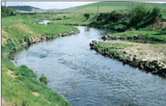
Narrowing increased velocities and created riffles used for fish spawning
