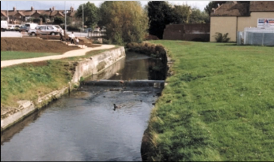
The river and weirs before construction
