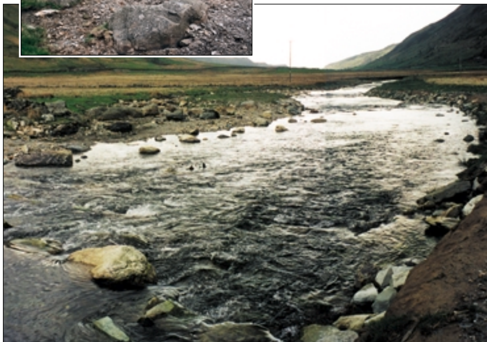
Restoration of boulder cascade, stepping stones and braided channel
