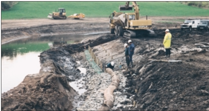
Figure 4.3.1 PROFILE OF LOG TOE REVETMENT
