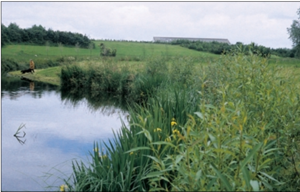
Willow spiling 2 years after construction
