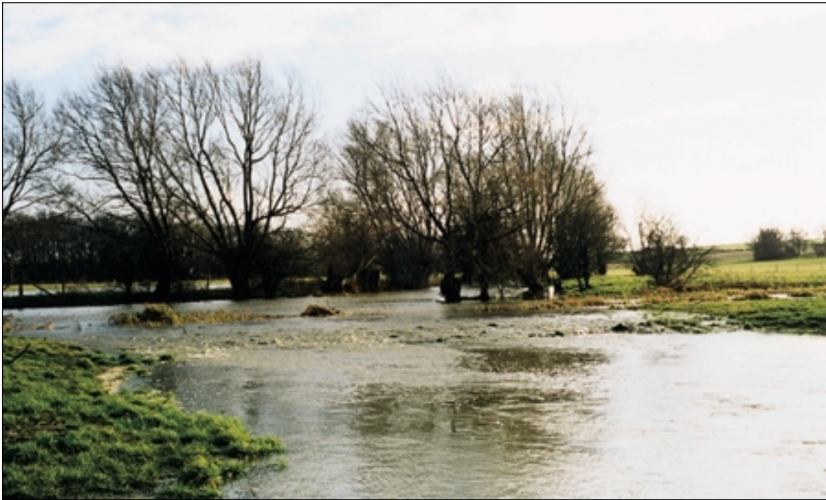
Spillway S2 in flood
