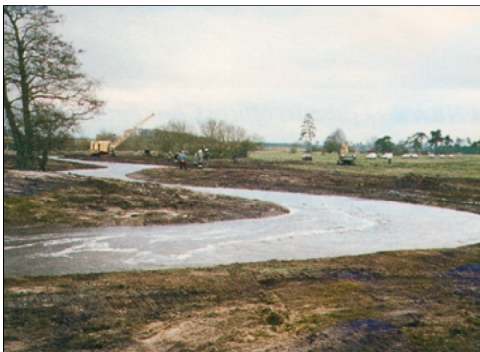
After reconnection to the river
