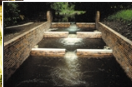
Mill weir and replacement fish-pass
