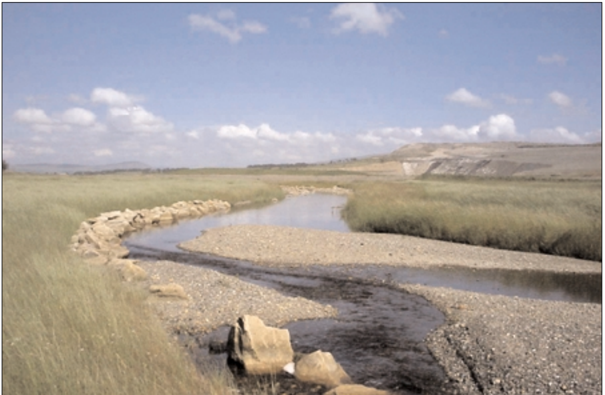
The rip-rap is still very evident but the in-river form is developing well
