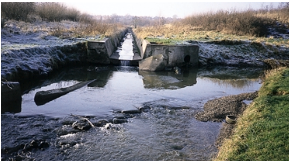
Yardley Brook – entering the River Cole. Before works
