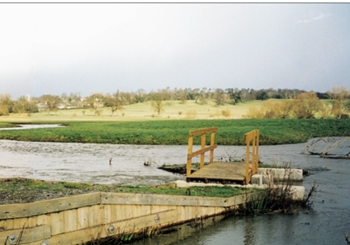
Flood filled channel downstream of bifurcation weir
