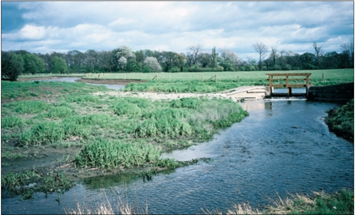
Spillway alongside bifurcation weir – April 1997
