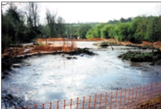
Dewatering – April 1995. View from inlet channel
