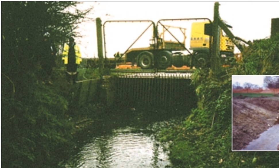
View of headscreen prior to removal
