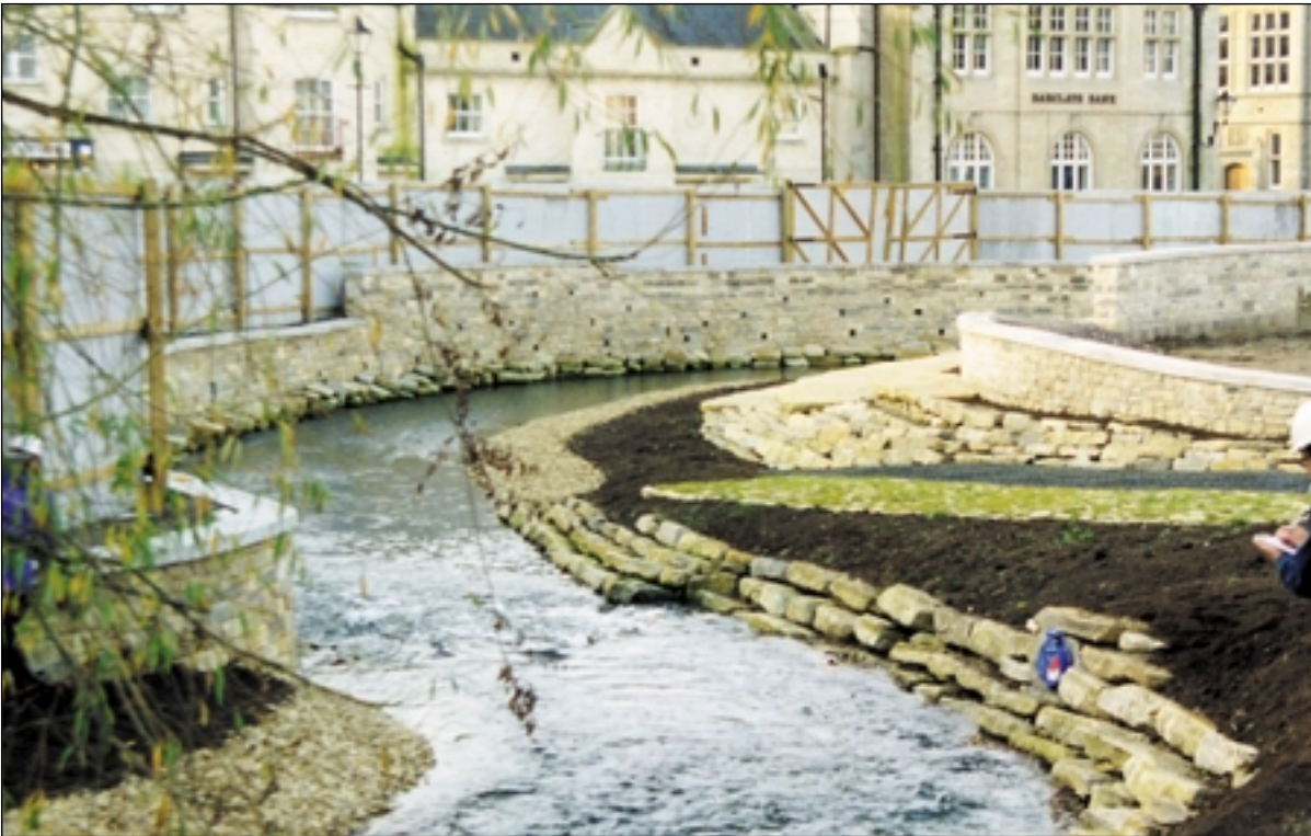
View of Section A (fig 1.5.3) on completion
