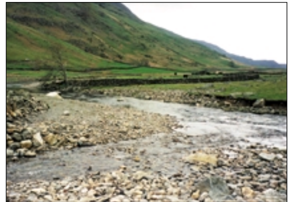
Restored bed levels and bank profile
