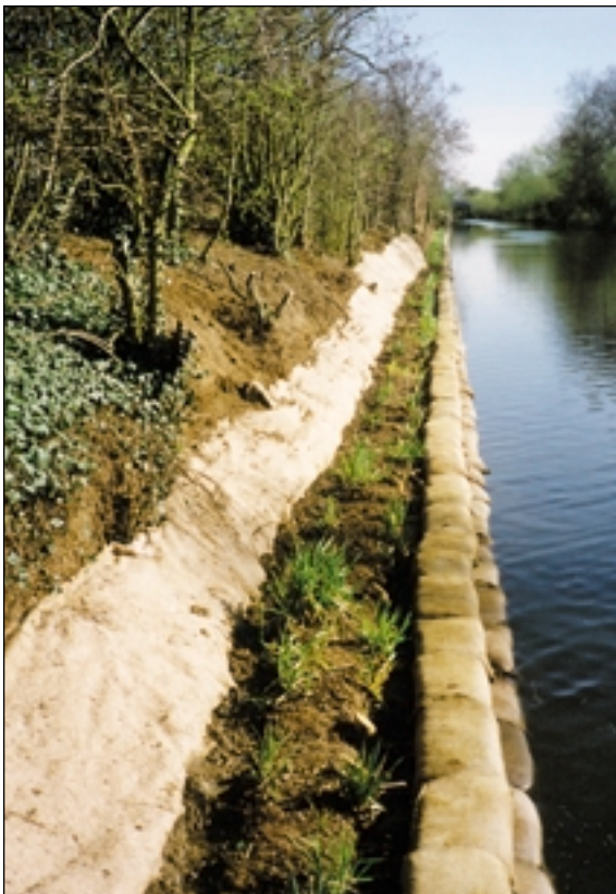
Flax mat secured, planted coir rolls installed and voids backfilled
