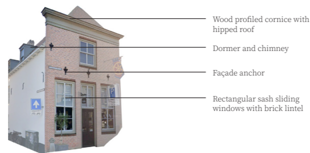
Figure 9. Botermarkt 22 Heusden, showing rectangular sash windows, façade anchors, dormers, wood profiled cornice and gabled roof (Google earth, 2026c, Heusden)
