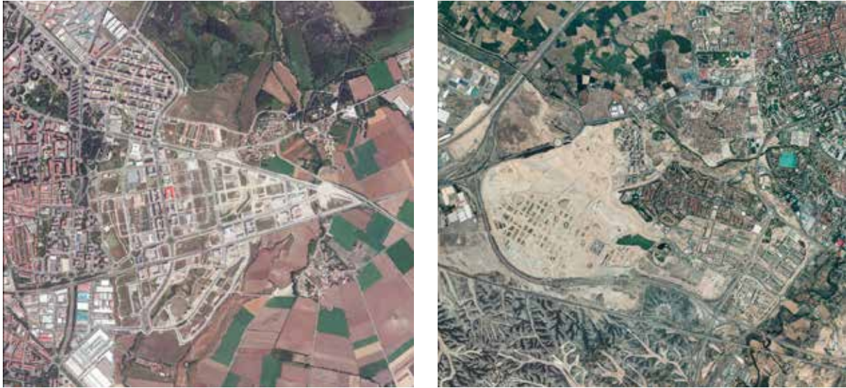
FIGURE 3 Aerial images of Vitoria outskirts —Salburua—, left, and Zaragoza outskirts —Arcosur—, right
