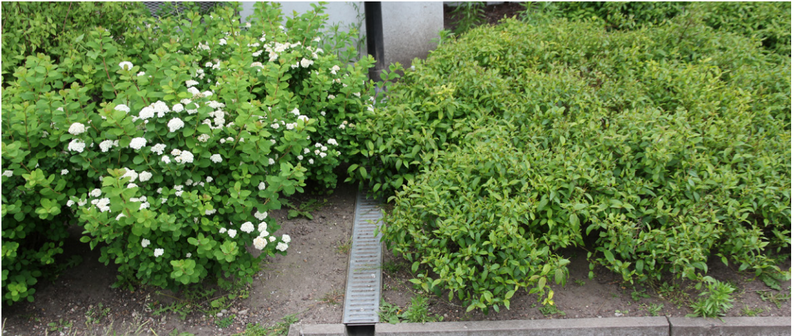
Storm water runoff from downpipes is diverted to water drop gutter.
