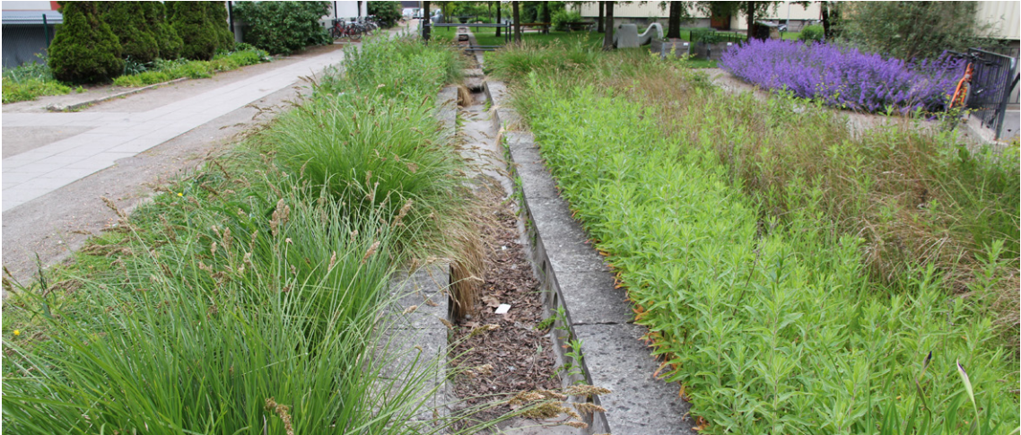
Concrete drainage canal with a mini-wetland for storage
