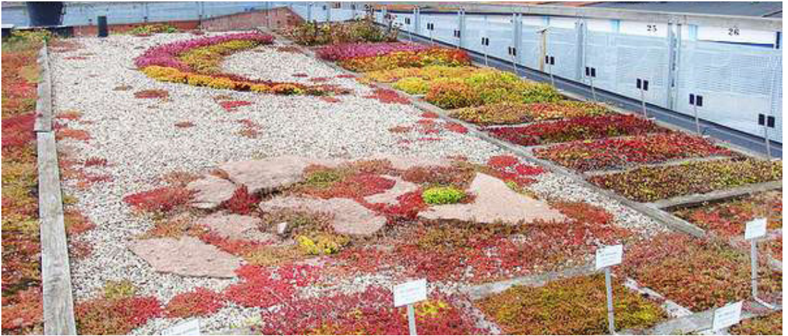
Botanical green roof garden: composed of different soil mixtures, plant mixtures, slopes.
