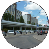
Metroline & Parking area (Commuting traffic problem)
