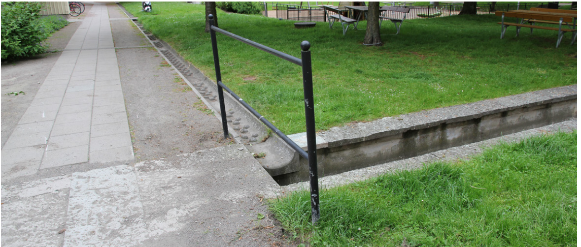
Water drop gutter end in concrete drainage canal
