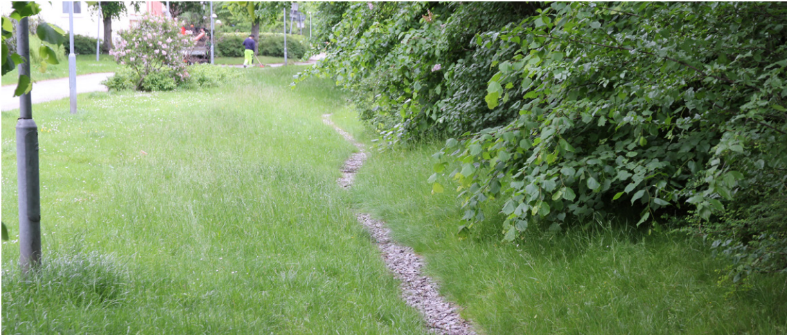
Swale in lower part of Lönngattan Drainage Corridor
