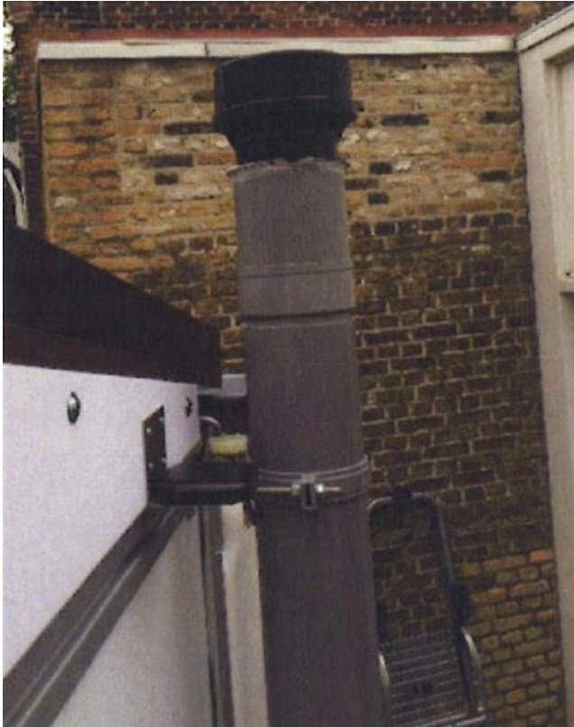
Figure 3-21 Granular activated filter for odour control in experimental eSOS Smart Toilet (Photo: J. Čurko)
