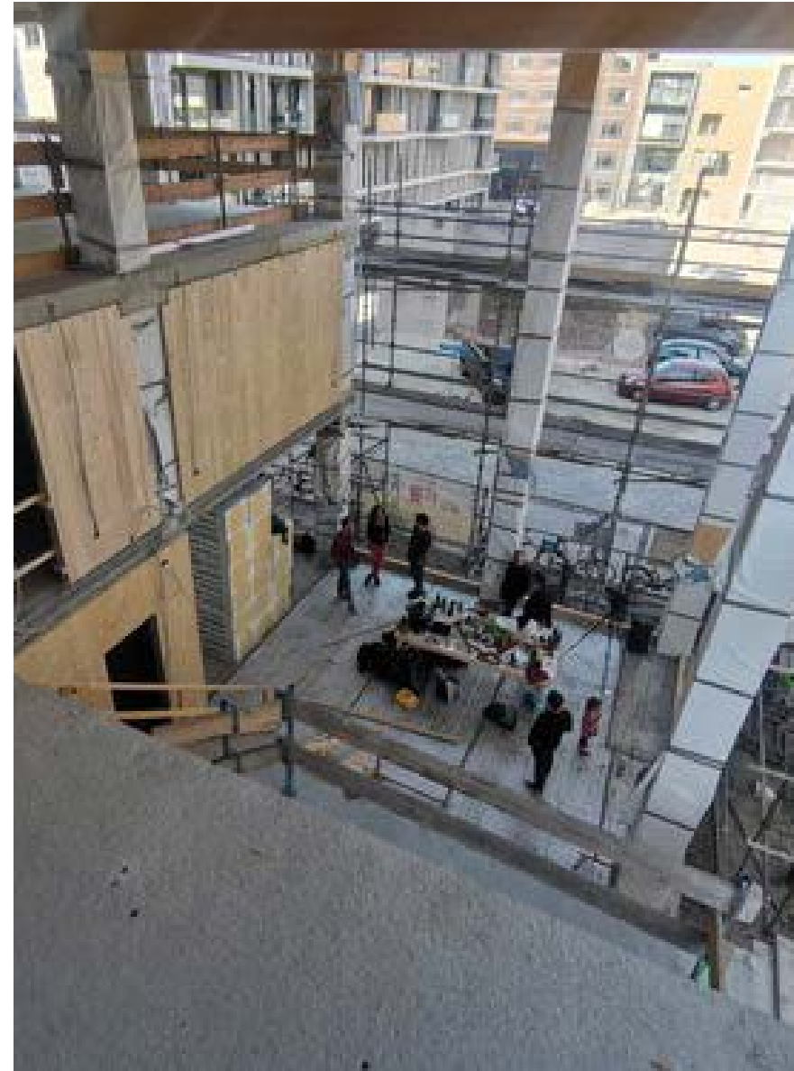
Image 2.7. Erik Loots (2022). De Warren under construction [Photograph]. https://dewarren.co/
