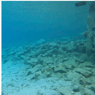
zone 3 | north pier break water
