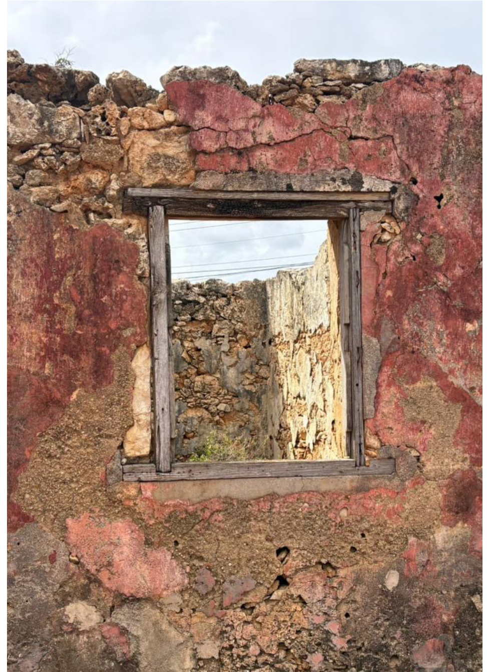
wooden lintel, stone wall and plaster finish | by author (2026)
