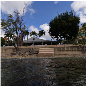
zone 1 | runoff stains on the boulevard
