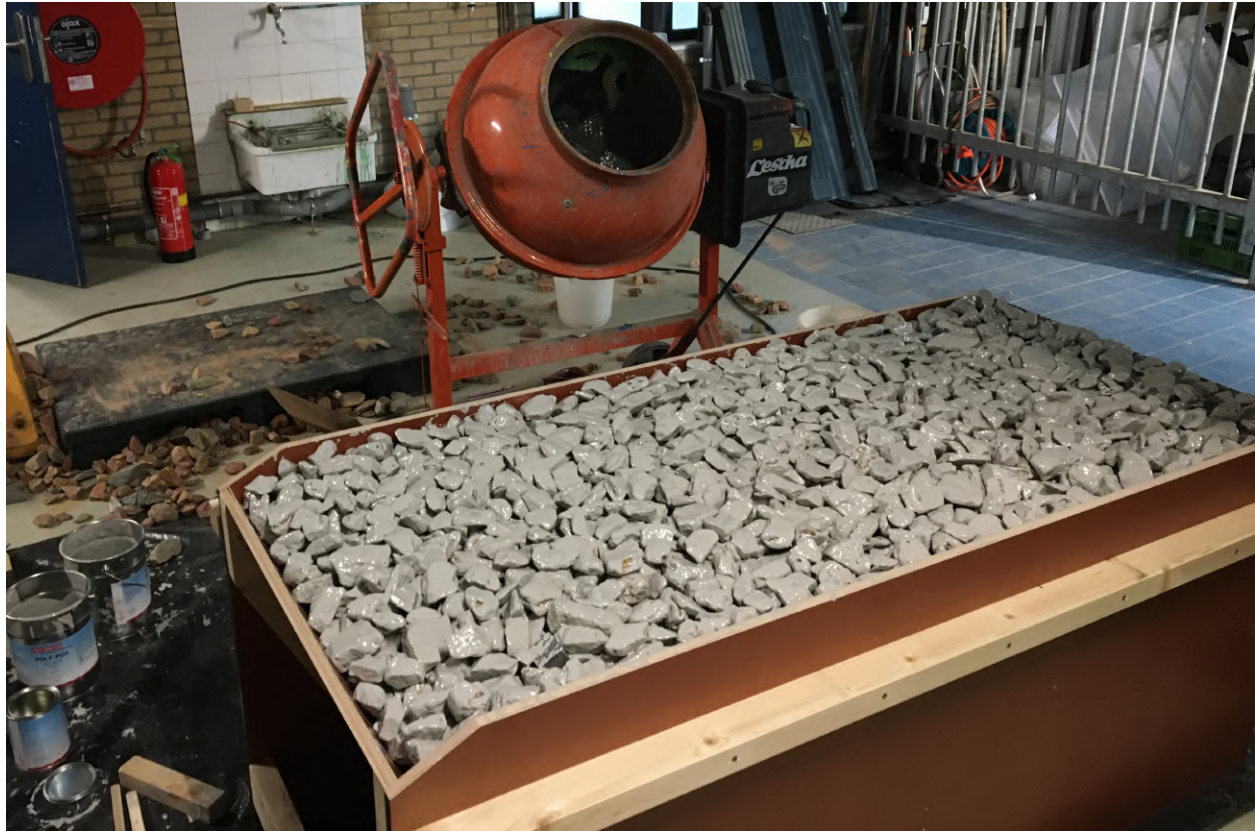
Figure C.2: Rigid breakwater after all the stones are thrown in to the mold.
