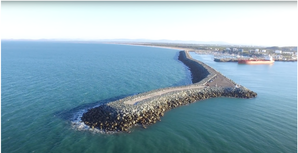
Figure 1.1: Conventional rubble mound breakwater. Location: Mackay (Australia)
