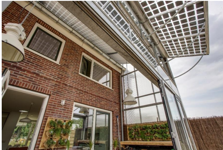
Fig. 11: The south side of the prototype house, featuring the integrated glasshouse
