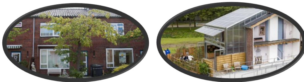
Fig. 95: Existing Honselersdijk house (left) and refurbished prototype (right)
