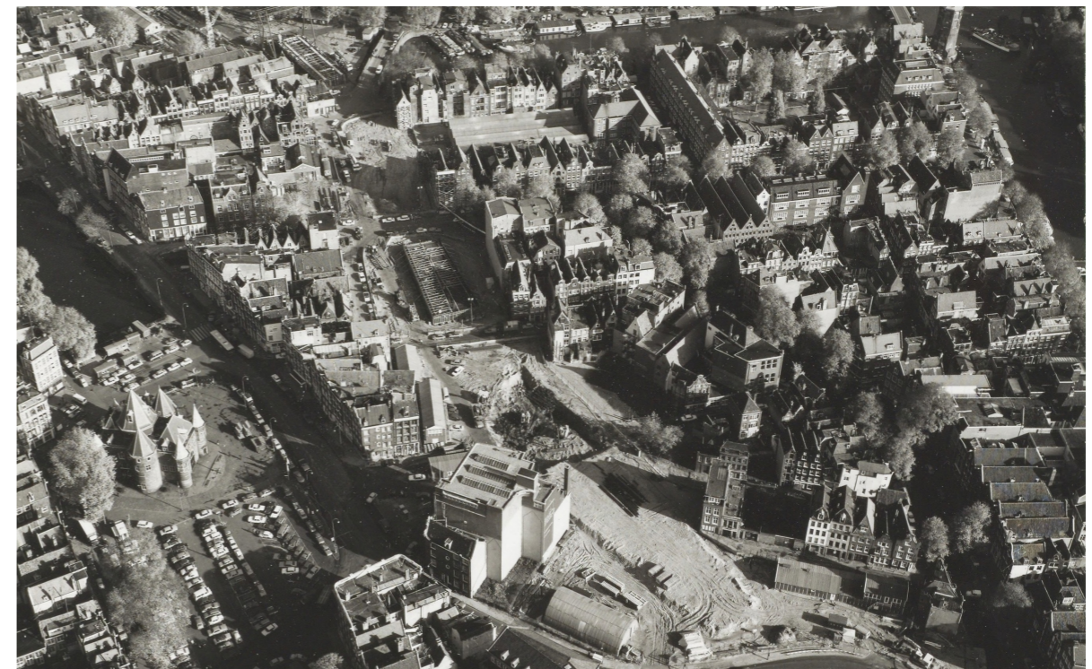
Figure 16a: Demolition for the metro around the Nieuw Markt (Stadsarchief, 1975a)
