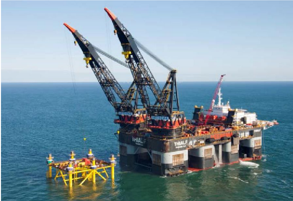
Figure 6: HMC's Thialf after installing a jacket
