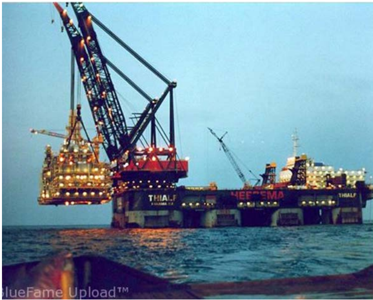
Figure 4: HMC's DCV Thialf lifting a deck platform
