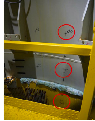
(b) Picture of the slip joint: the red circles refer to three sensing sections along the vertical direction.
