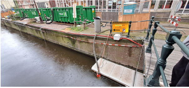
Figure 6. Test loading of historic quay wall along Rechtboomssloot in Amsterdam
