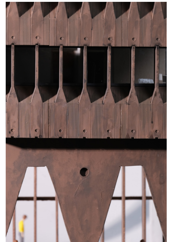
Figure 55 - Facade fragment model 1:25, showing facade soiling (Lars Haga, 2026)
