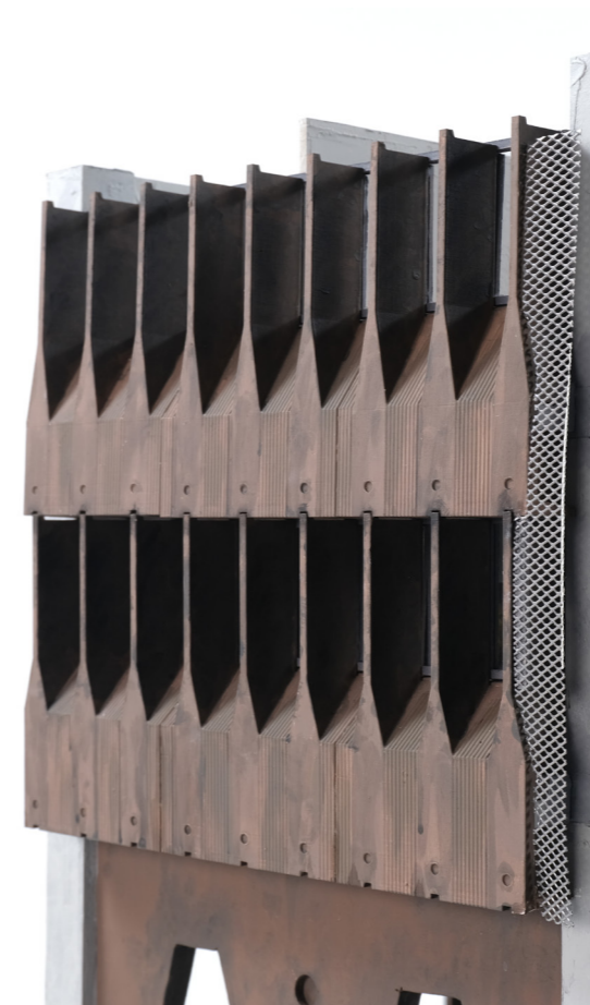
Figure 54 - Facade fragment model 1:25, showing facade soiling (Lars Haga, 2026)
