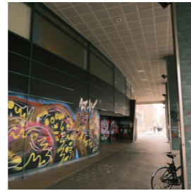
Figure 06 - New ground floor facade
