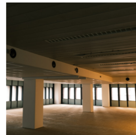
Figure 14 - Lowered ceiling with vents
