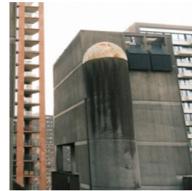
Figure 11 - Water streaks
