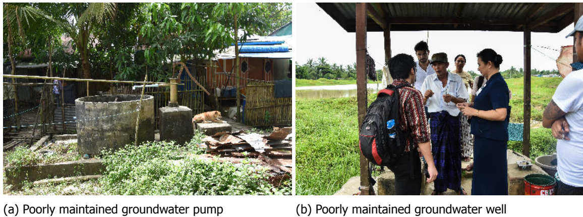
Figure 6.8: Out-of-order water facilities due to poor maintenance and operations
