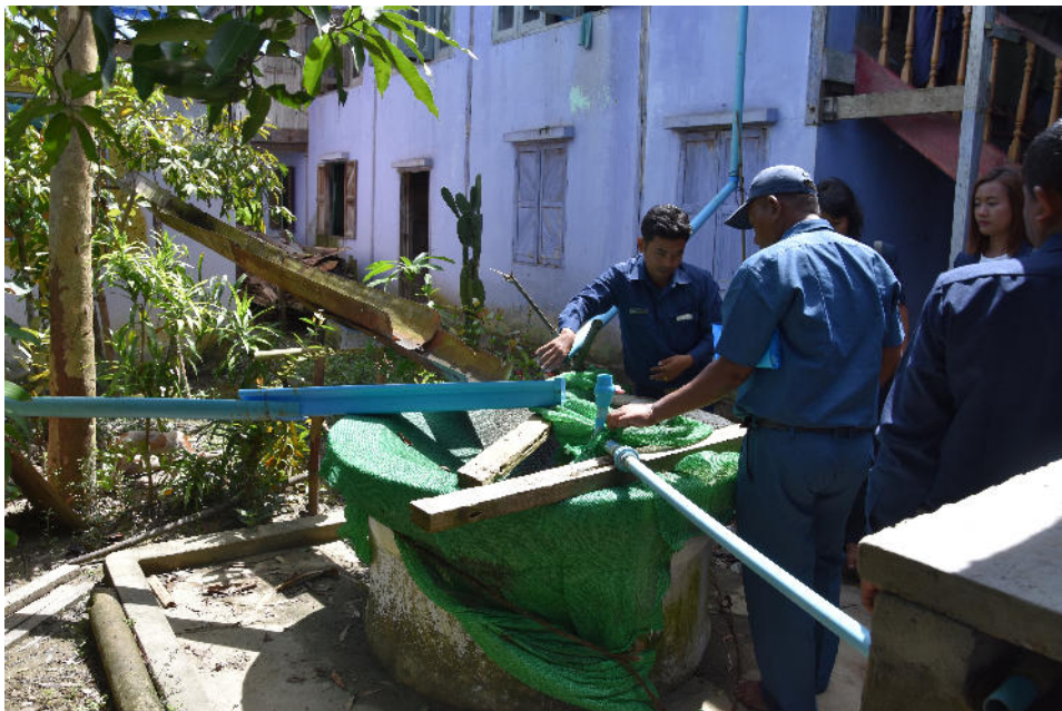
Figure 7.1: Covered rainwater collection point
