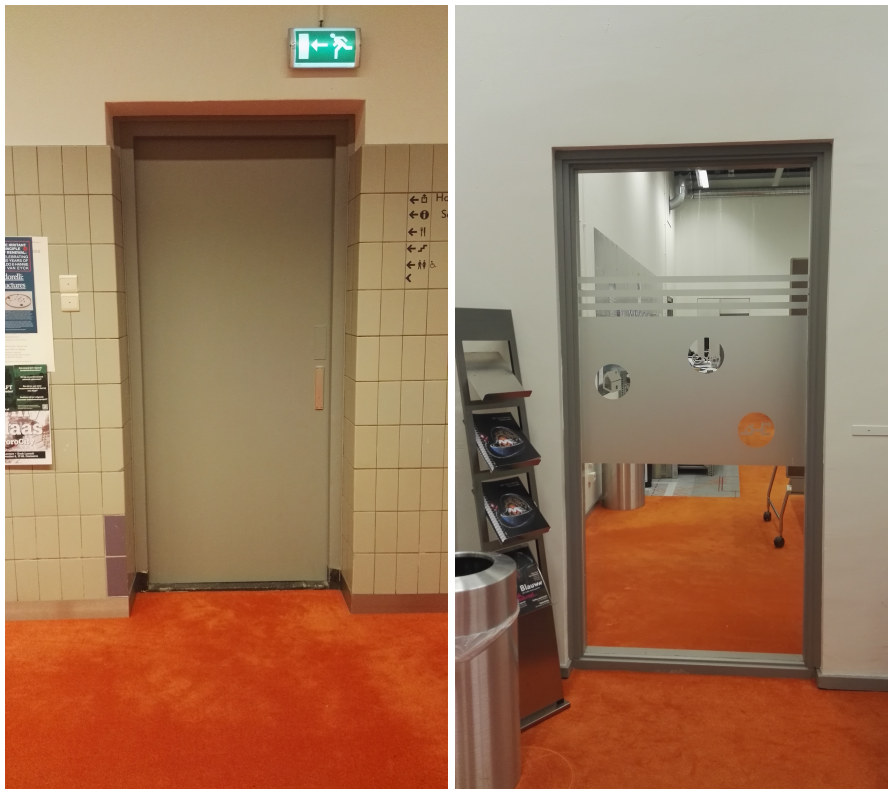
(a) A permanently closed door (b) A glass pane in place of a door frame
