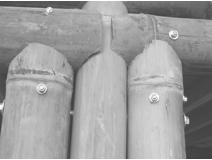
Bamboo Connections Bolted
