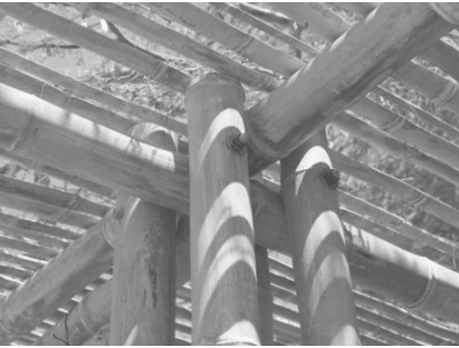
Bamboo Connections Bolted
