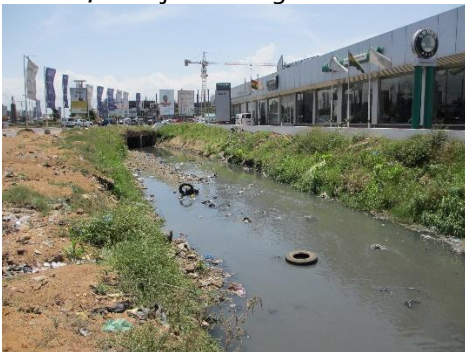
Figure 43 Drain Graphic Road (Author's source, 2016)
