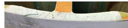
Figure 4.26: Detailed picture of the spar cap. Picture provided by the Re-Wind Network
