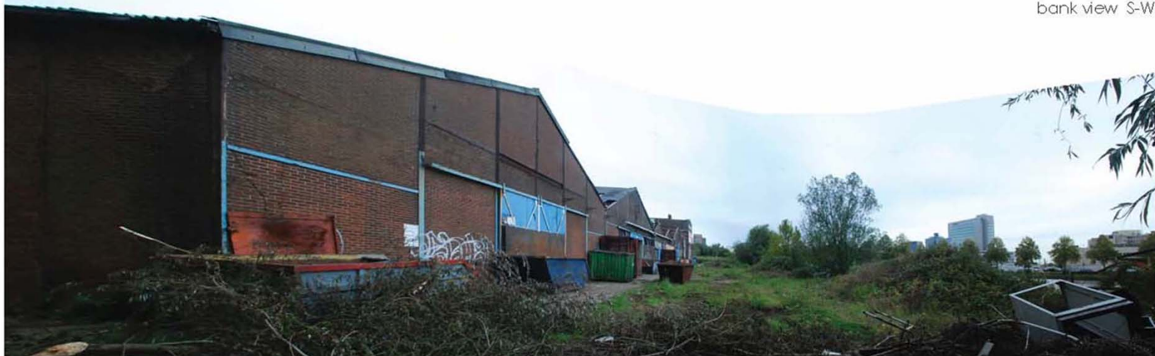
bank view N-W
