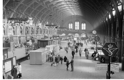
Copenhagen central station
