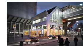
Maashaven metro station, Rotterdam, Netherlands Area: 2882m 2 Capacity: 12400p/day
