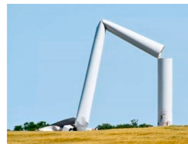
(c) support structure (tower) [27]
