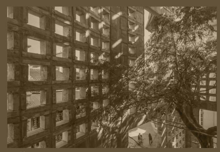
**Transition** Porous facade allowing filtered light to pass through
