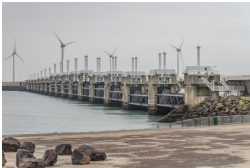
Tab S9. Maeslant barrier (The Netherlands)
