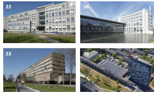
Figure 4: TU Delft campus buildings listed for adaptation. Van den Dobbelsesteen, A. (2022). Climate Design & Sustainability [Slide show; Research Lecture]. Brightspace. https://brightspace.tudelft.nl/d2l/le/content/503093/viewContent/3089449/View
