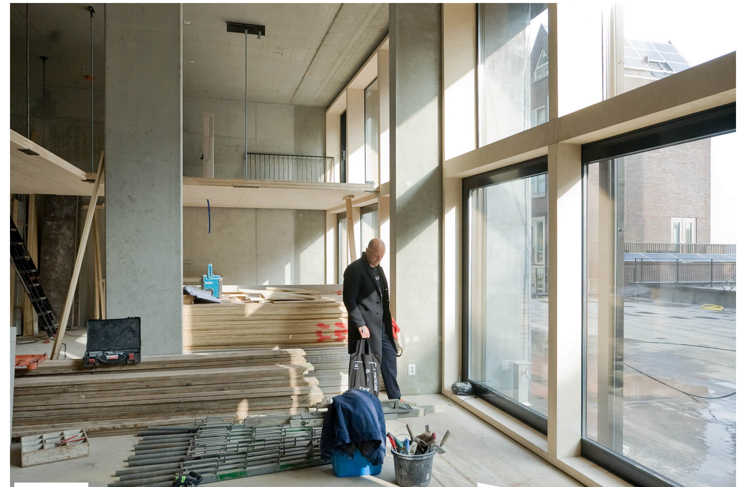
Figure 50. CLT mezzanine during construction. (Source: Marc Koehler Architects, n.d.)
