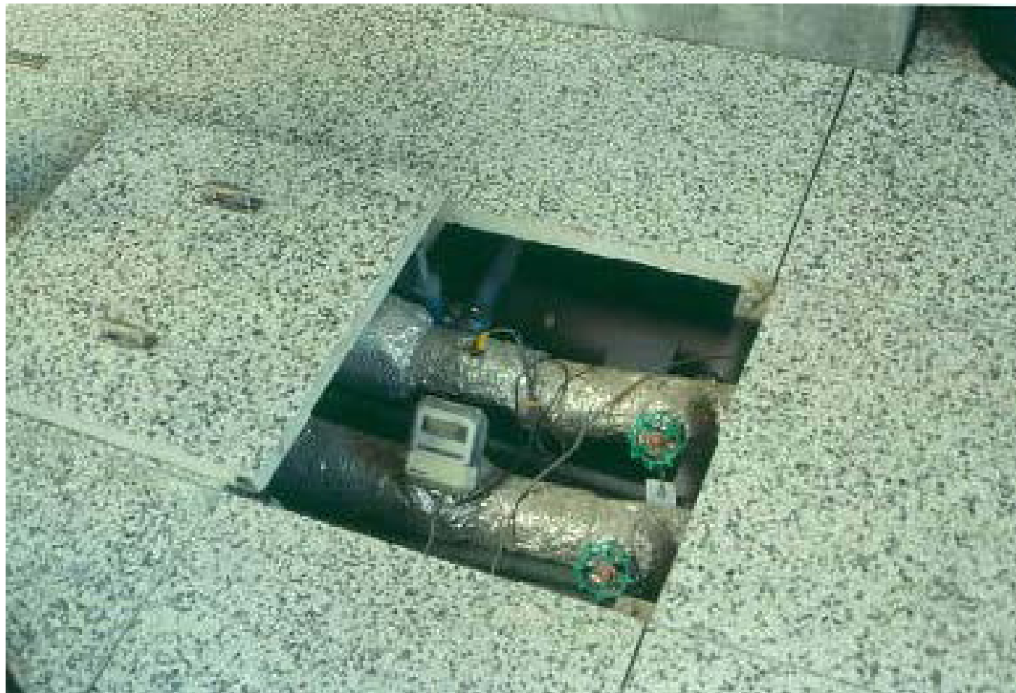
Figure 101. Raised floor with removable top layer. (Source: Kim, 1993)
