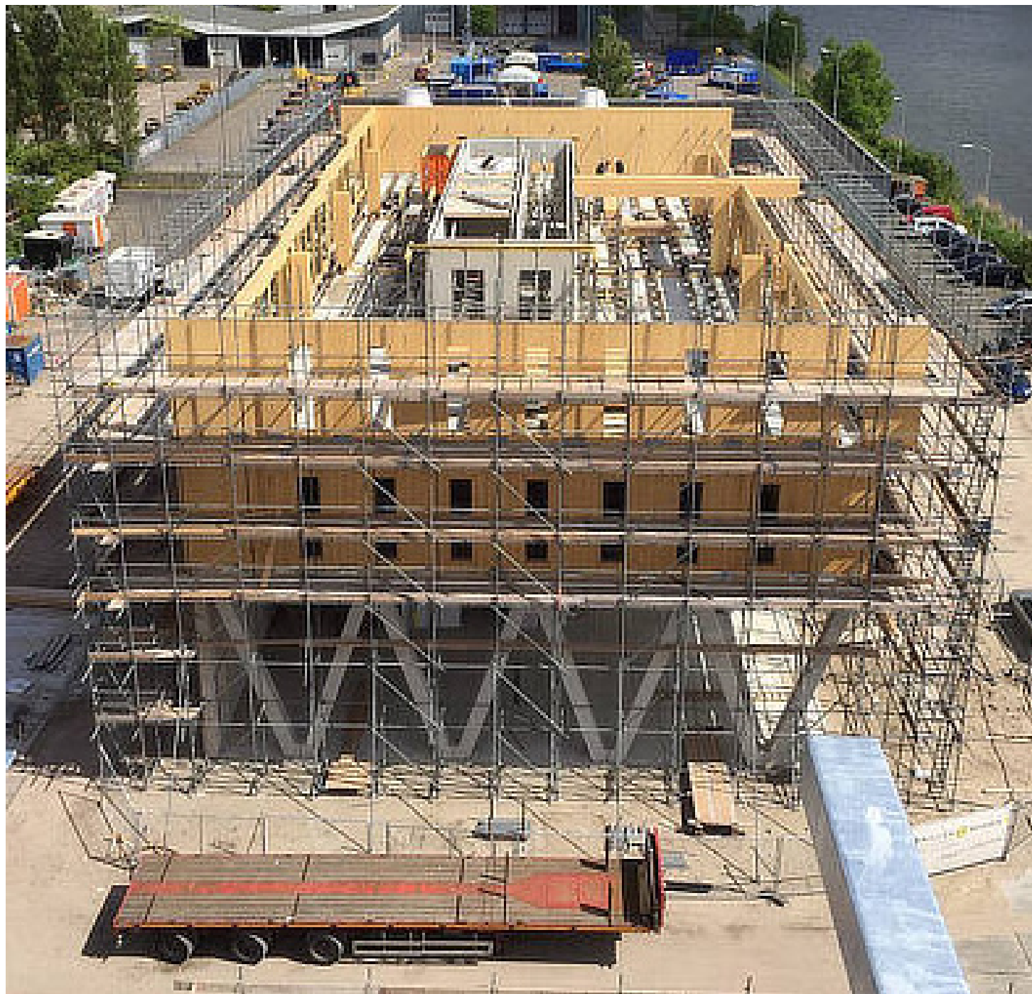
Figure 8. Column and beam structure with stablee core as seen on site. (Source: Arketipo Magazine, 2023)
