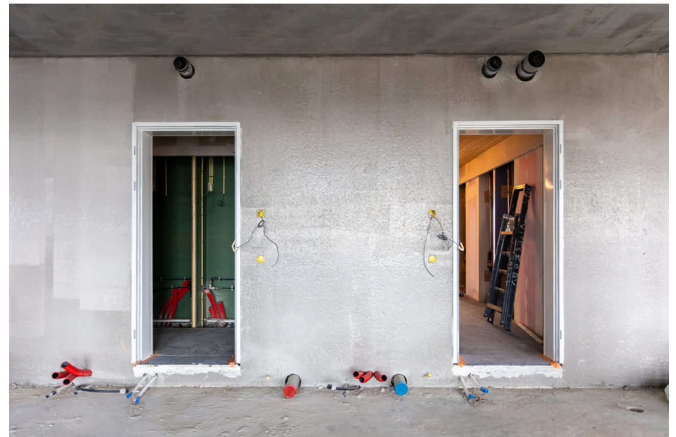
Figure 60. Capped off delivery of piping, example from TOPUP. (Source: Frantzen, 2021)
