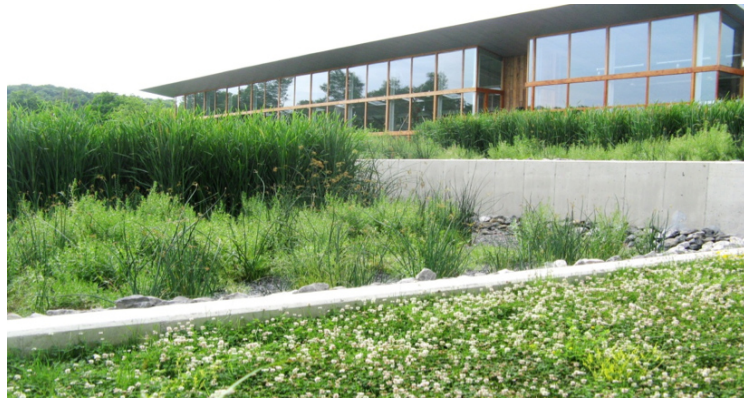
Figure 31 - Typical Subsurface flow CW
