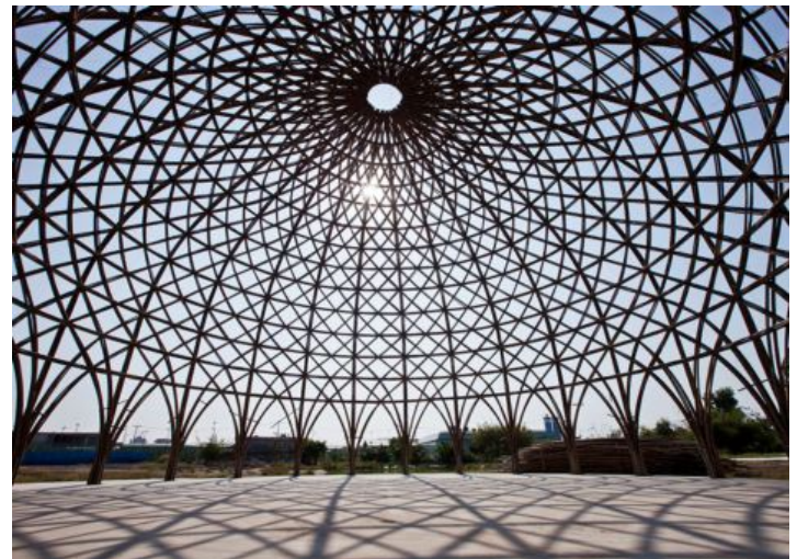
Figure 22 – Ribbed dome with lamella dome
