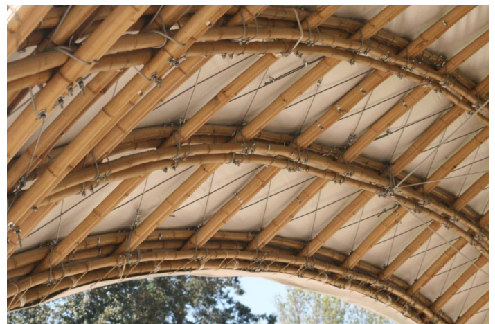
Figure 20 - structural joint detail bamboo pavilion
