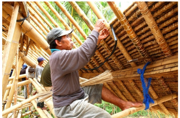
Figure 24 - Thatch with integrated horizontal laths
