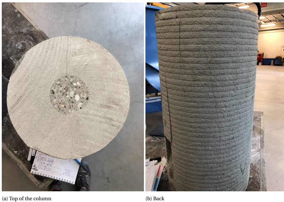
Figure 9.4: The cracks of the concrete printed element, after it failed
