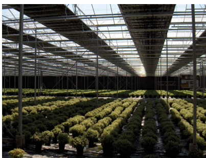
Figure 1.7: Sun blocking screen to control the amount of sunlight that enters the greenhouse [64]
