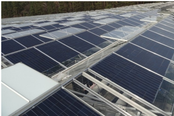
Figure 3.5: c-Si modules integrated in greenhouse roof by replacing glass [135]
