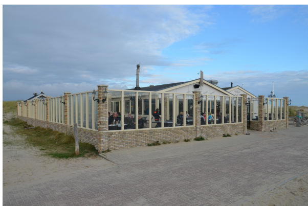
Figure 4.2: Current building on building site
