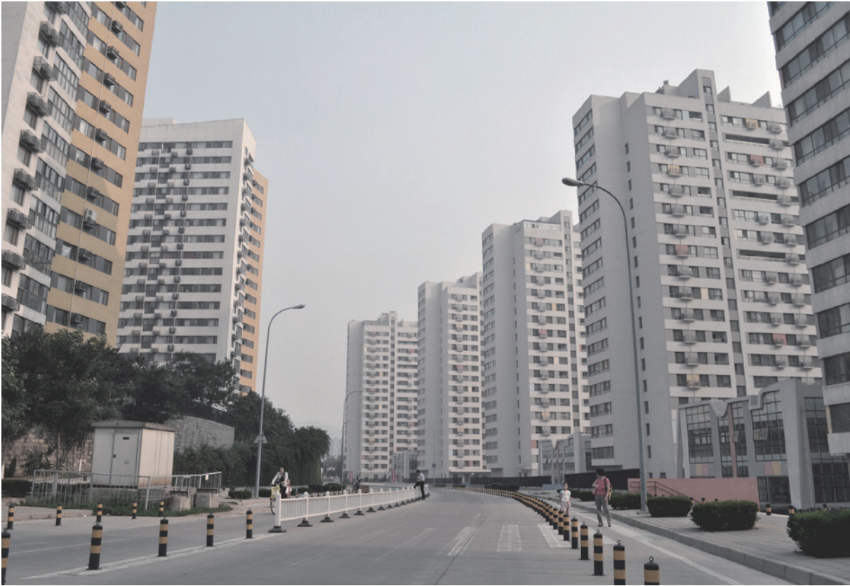
figure 2.2.3 The ubiquitous high-rise superblock in China
