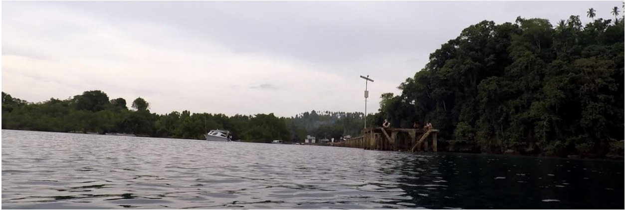
Figure 70: Site visit pier on the right and mangroves on the left
