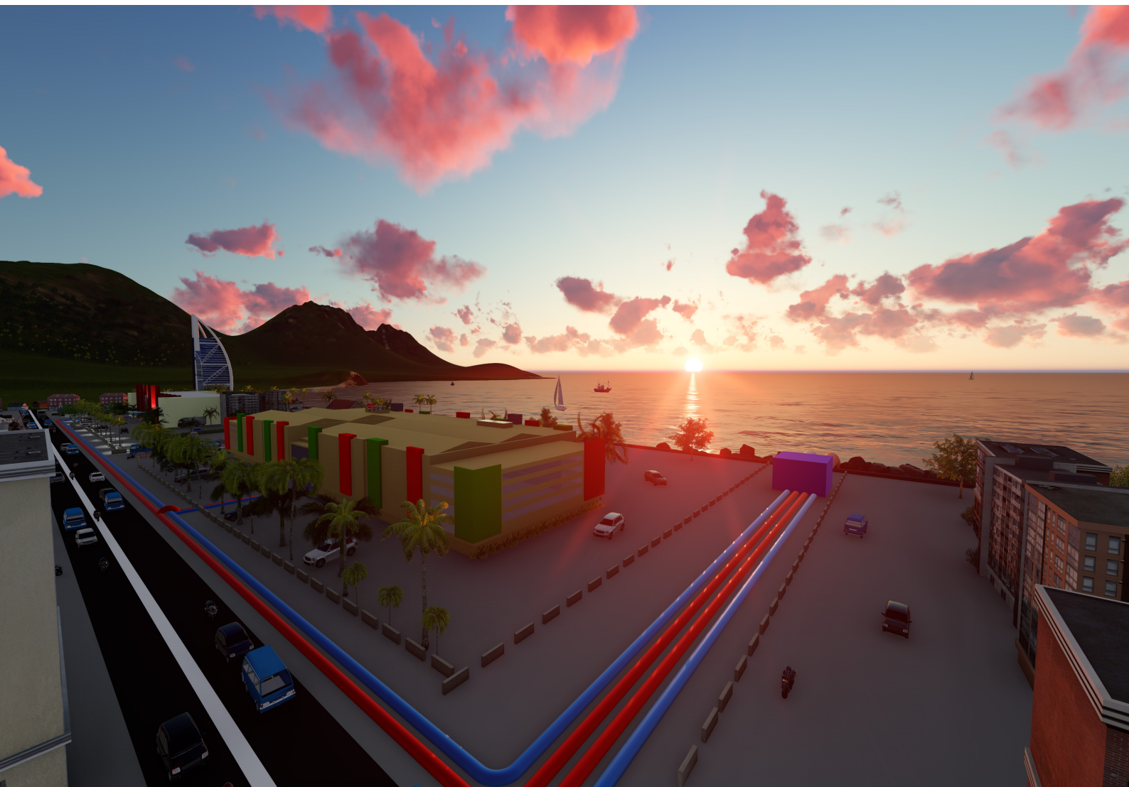
Figure 57: Artist impression of Manado bay (Note: in reality the onshore pipes are buried and the sizes are disproportional for visual representation)
