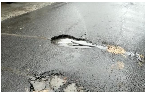
Figure 32: Broken water pipe
