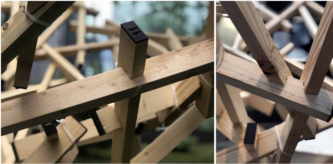
FIG. 5.19 Top: The final prototype with 78 reciprocal elements varying in size ranging from 500mm to 1700mm Bottom: Close up of the connections.
