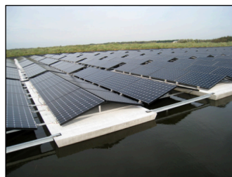
Pontoons with metal structures
